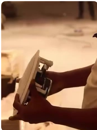
Installing a ceiling speaker
